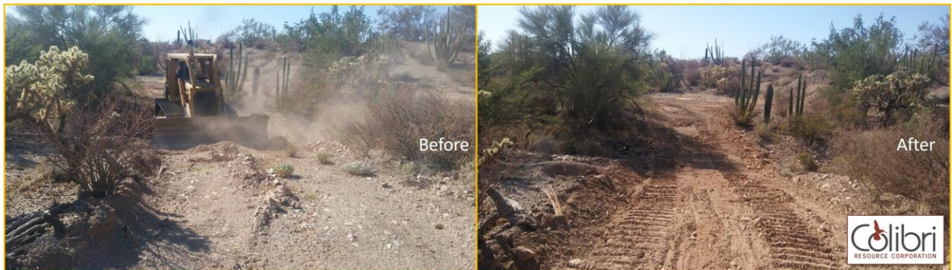
Illustration 2 – Road Repairs at Evelyn Gold Project
